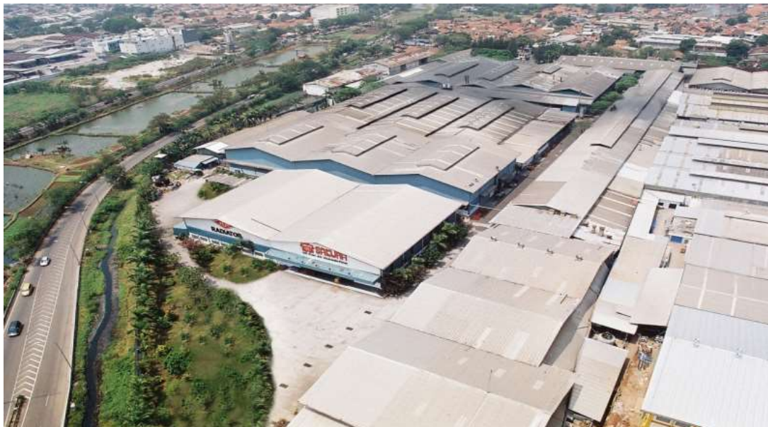
Kapuk Plant (Radiator Facilities)
